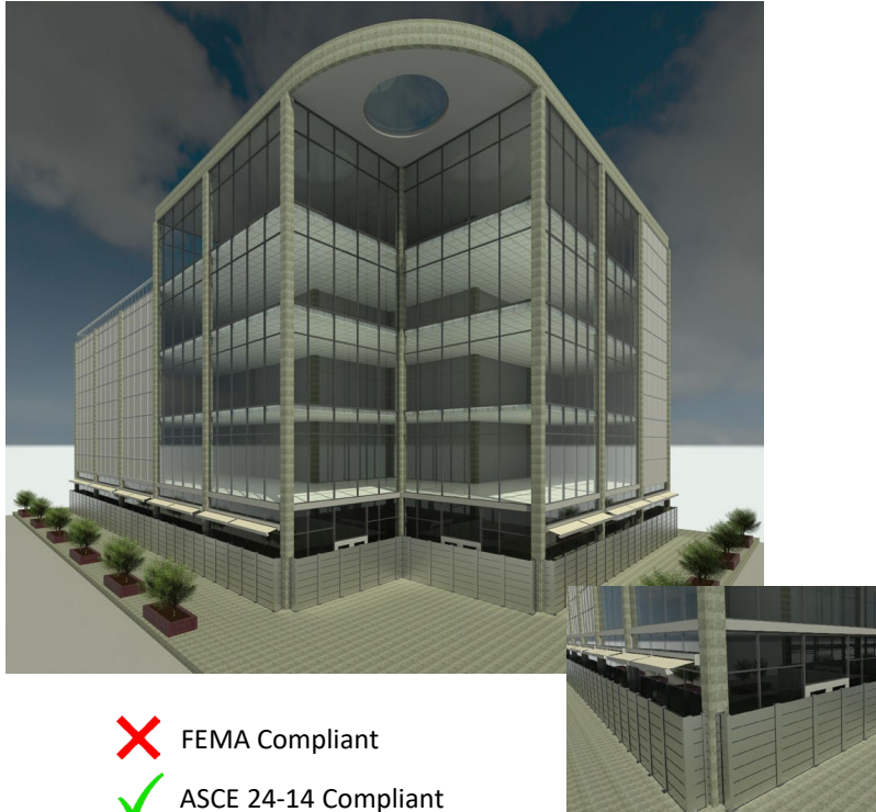
Non-floodproof Window and Wall System with Deployable Flood Barriers
