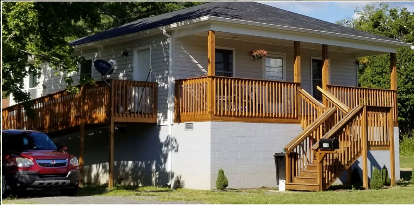
Elevated Structure (with flood vents)
